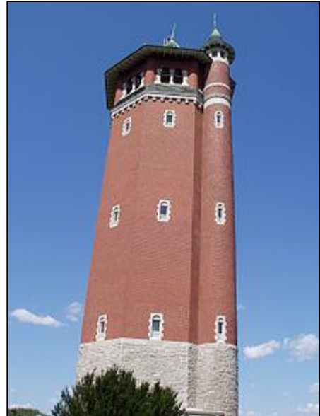
High Service Water Tower
